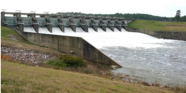
Toledo Bend Dam, Hydropower, TX and LA
