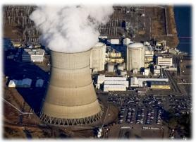
The ANO site consists of two pressurized water nuclear-powered electrical generating plants; Unit 1 (a Babcock and Wilcox Nuclear Plant, rated at 836 MW) and Unit 2 (a Combustion Engineering Nuclear Plant, rated a 993 MW).
