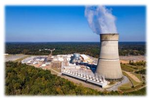
The Grand Gulf Nuclear Power Plant ("GG") consists of a General Electric Manufactured Boiling Water Reactor with a capacity output of 1,443MW, making it the largest commercial nuclear power plant in the United States. GG, located in Port Gibson, Mississippi provides approximately 33% of its power to the State of Arkansas. Recently, GG experienced a forced outage requiring the plant to be out of service for approximately five months. The Arkansas Attorney General has engaged CTC to perform
